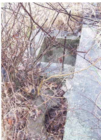
Decaying spillway.
