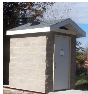
New pit latrines have been completed at Whitham Woods, Lamson Woods and at the intersection of Cedar View Trail and the Loop Trail.
